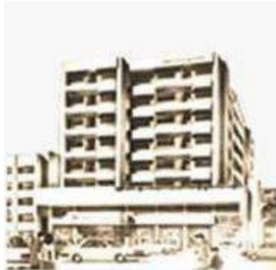
SOLER TOWER RESIDENTIAL, MANILA
